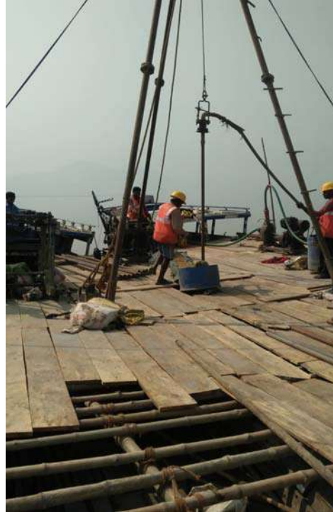
Boring in Progress (RBH-01)
