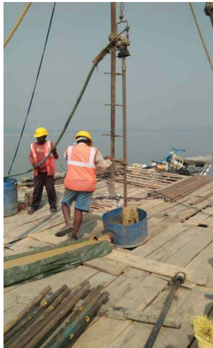
Boring in Progress (RBH-01)
